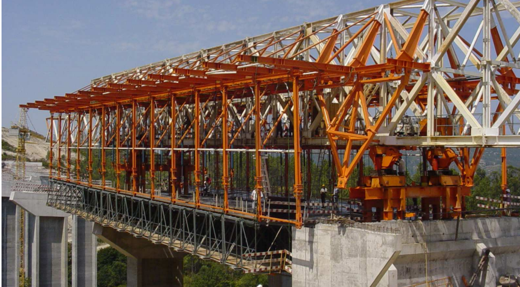
Figure 8: K launching gantry
