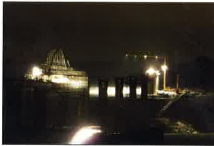
Fig. 3: Bridge across the Hostovsky Creek Valley (night works)
