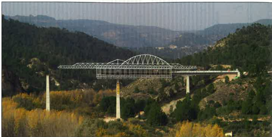
Fig. 1: Rio Cabriel Bridge, Spain
