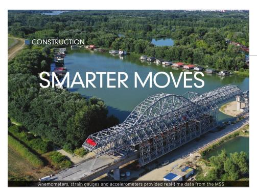
An enhanced monitoring system for movable scaffolding systems has been tested during construction of a highway bridge in Slovakia, write Pedro Pacheco, André Resende and Filipe Magalhães
