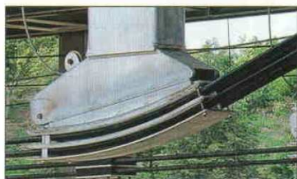
Fig. 13: (a) Deviation saddles in concrete pouring position (b) and in launching position
