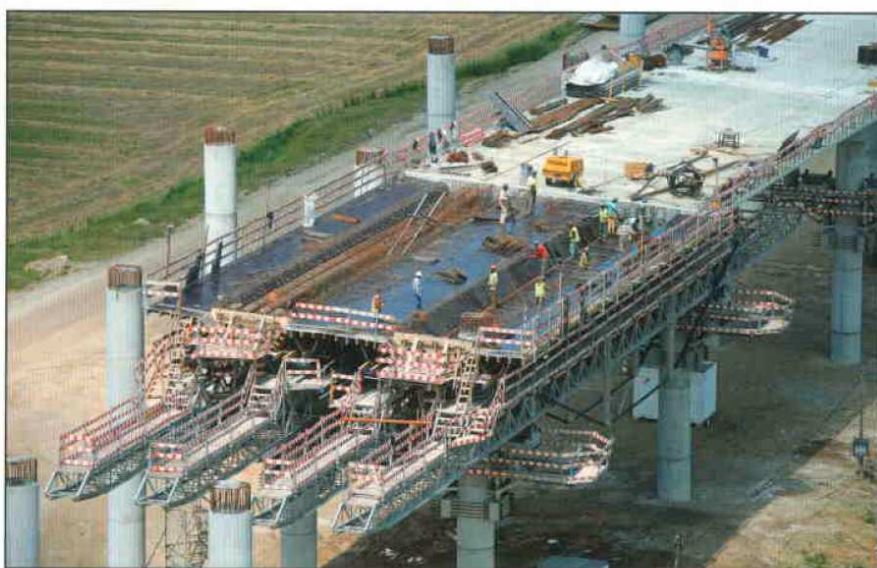
Fig. 16: General view of on site operations over OPS movable scaffolding system
