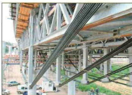
Fig. 12: (a) Cables and deviation shores in concrete pouring position (b) and in launching position
