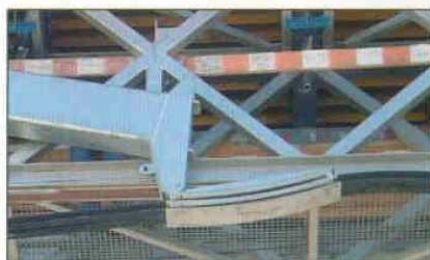
Fig. 13: (a) Deviation saddles in concrete pouring position (b) and in launching position
