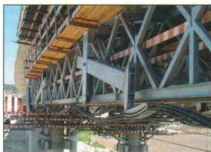
Fig. 12: (a) Cables and deviation shores in concrete pouring position (b) and in launching position
