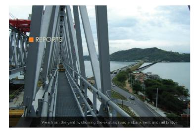
When Bd&e visited the site in November last year, work had progressed from the in situ construction to the use of the Berd launching gantry, which can erect a 50m-long span in less than a week. In November work was about to start on the over-water span construction. Work on building one of the towers for the cable-stayed span had already begun the month before, with the second one just about to start.
