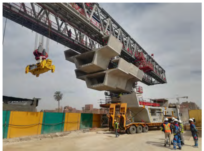
Figure 11: Transportation of segments from a truck
