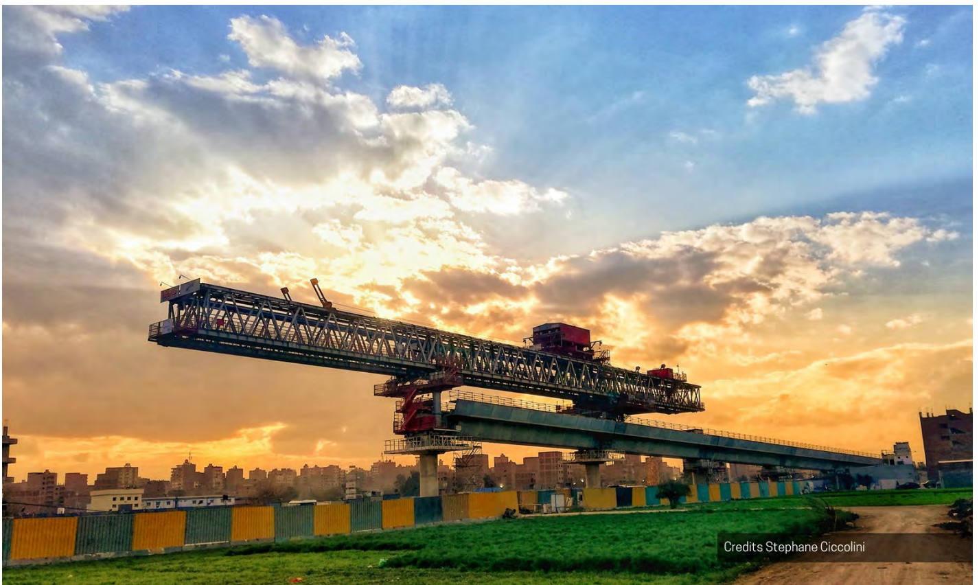
Figure 1: Launching Gantry in operation
