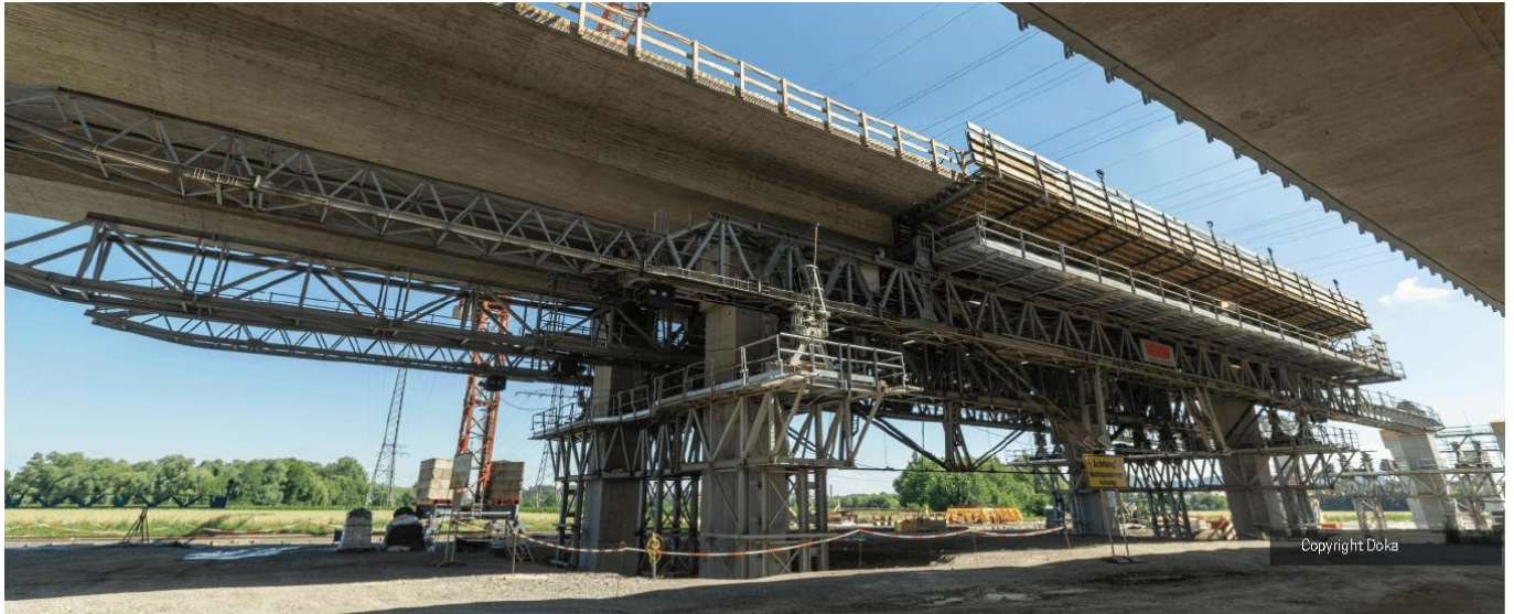
Figure 2: Underslung movable scaffolding system M38-I
