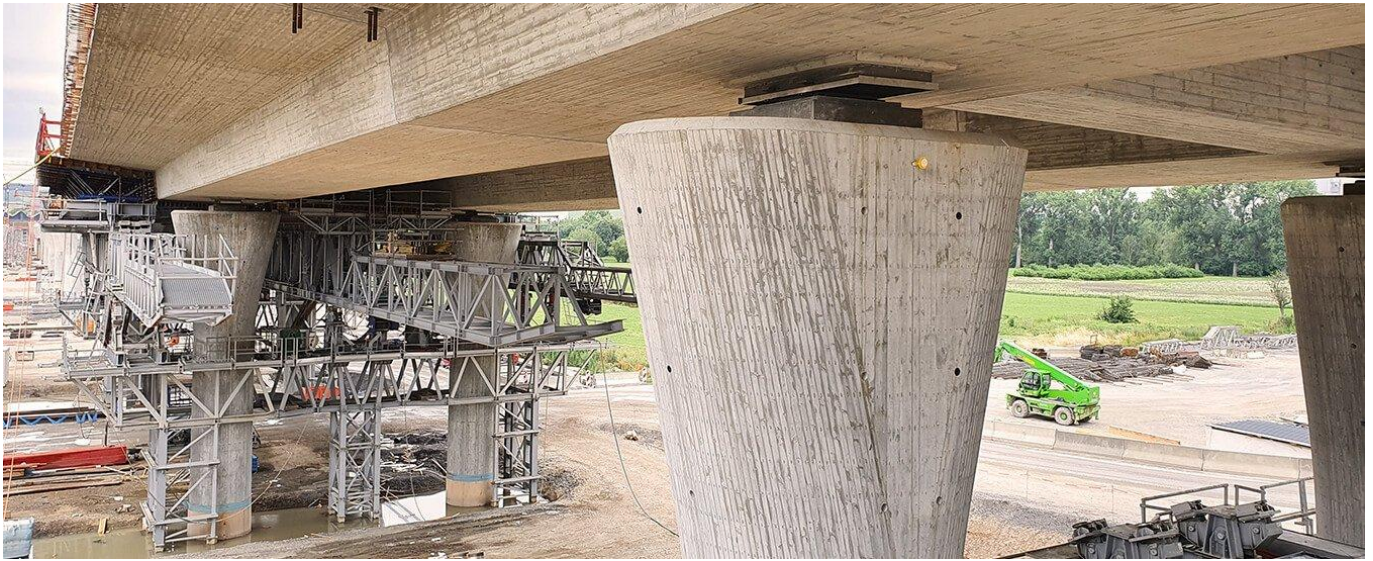
Figure 6: The MSS operating under the deck
